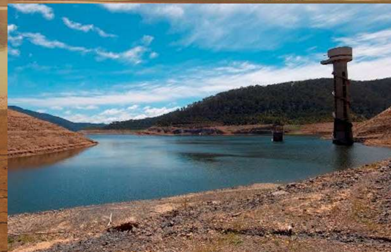
Thomson Dam, Melbourne's largest water storage, during the Millennium Drought
